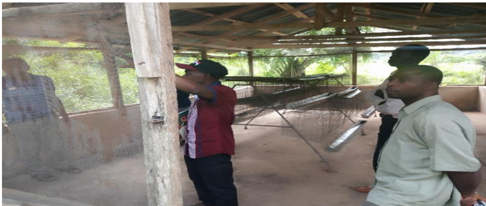
Figure 3: Renovated poultry pen at Mamu school.
