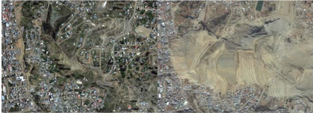
Figure 4: The 26 February 2011 megadeslizamiento, a big landslide that devastated large parts of the city of La Paz. Left: the area before the catastrophe; right: the area afterwards. (Photos courtesy of Gobierno Autonomo Municipal de La Paz [GAML])
