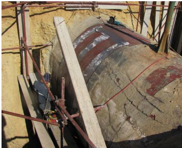
a) Preparation of the external pipeline surface
