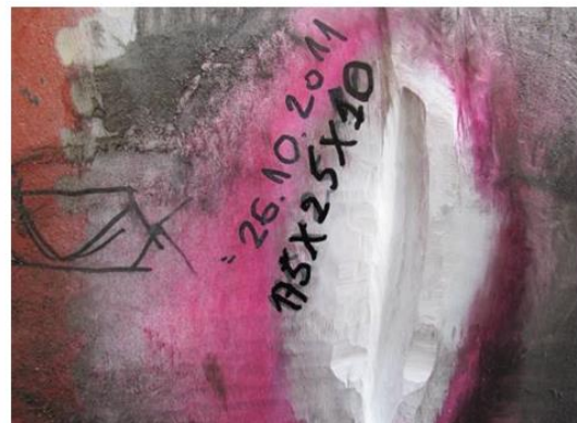
b) An area prepared for surface welding
