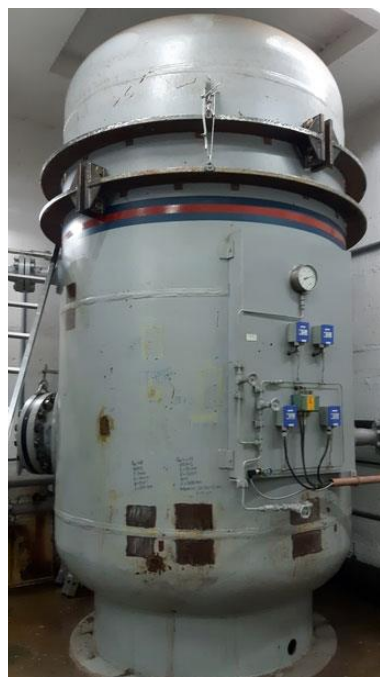
Figure 2. The pressure vessel 970, after repair with stiffener.
