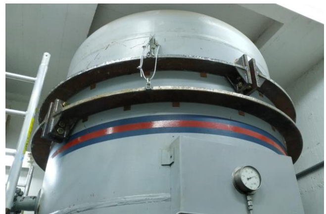
Figure 10. Details of the two-ring reinforcement solution.
