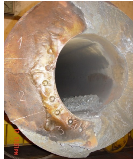
Fig. 4. Zone of through wall crack on the hollow shaft; zones 1, 2 and 3 represents crack growth front of the through thickness crack, and the rest of the surface was flame cut surface
