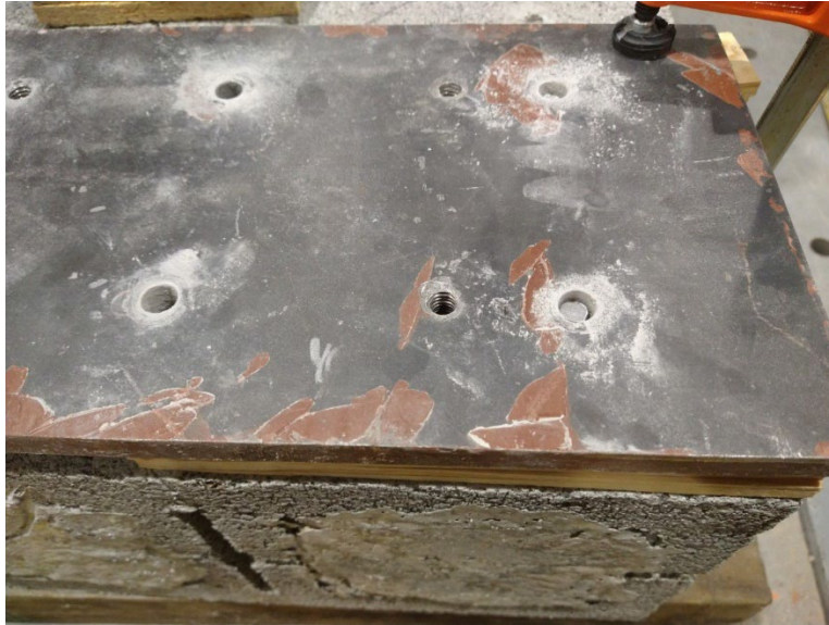
Figure 26. Threaded Rod Lined Up with Steel Plates
