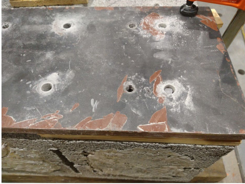
Figure 14. Steel plate overlaying inserted threaded rod
