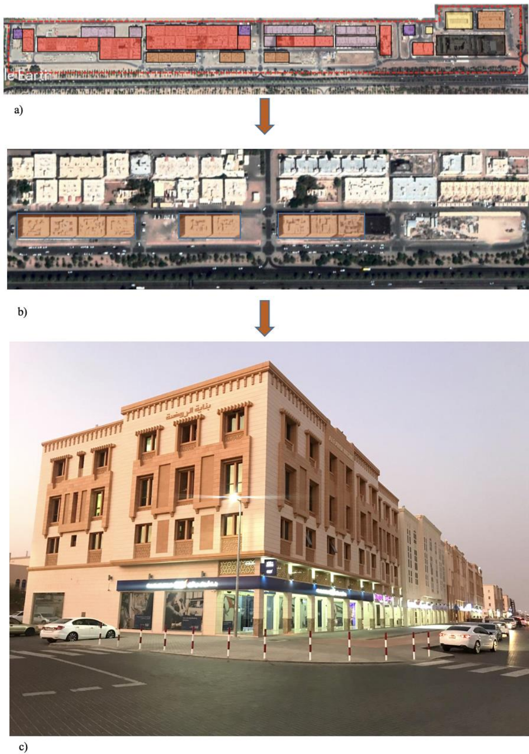
Figure 34: Mixed-Use Multi-Story Blocks (a, b, c) in Zone A (Google Earth Maps, 2019).
