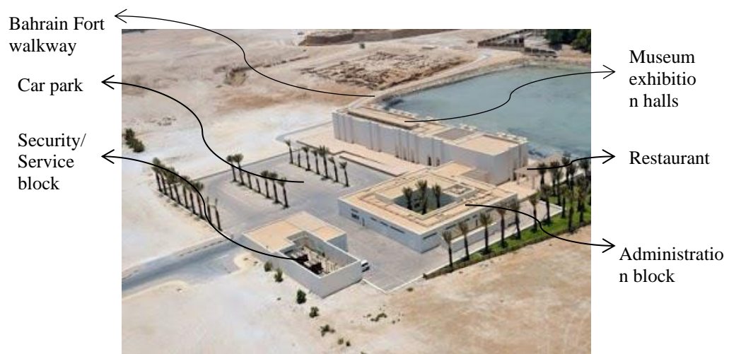
Figure 4.14: Qal'at Al Bahrain site museum aerial view and functional components
