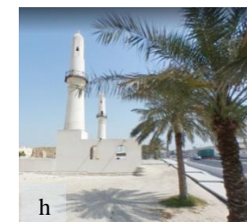
h Between the site and the main road – Looking east
