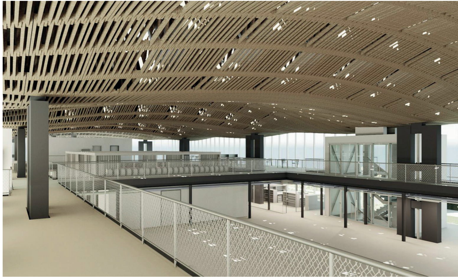
Fig. 8: Roof structure seen from the inside of the building.
