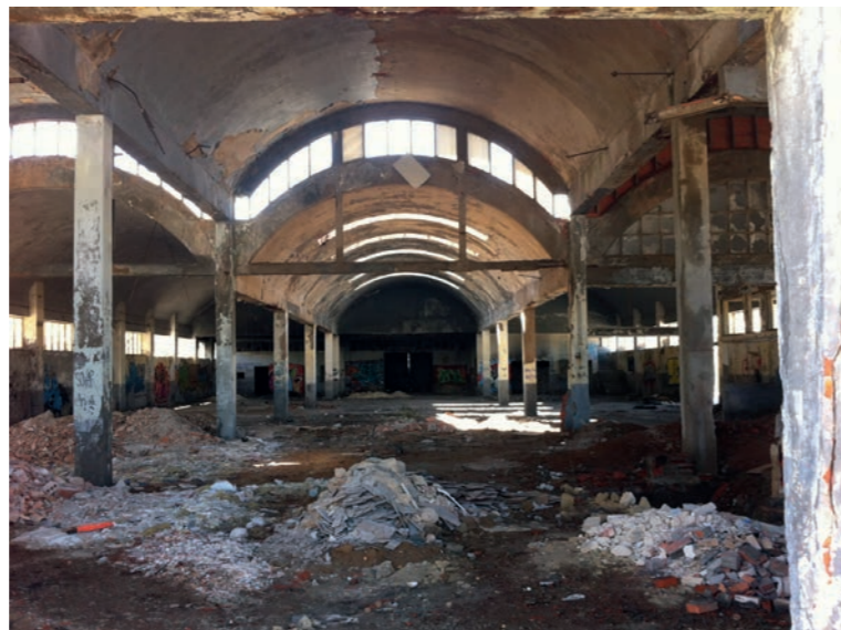
Fig. 3 Vitasal structure of three barrel. Photo by Gonçalo Canto Moniz
