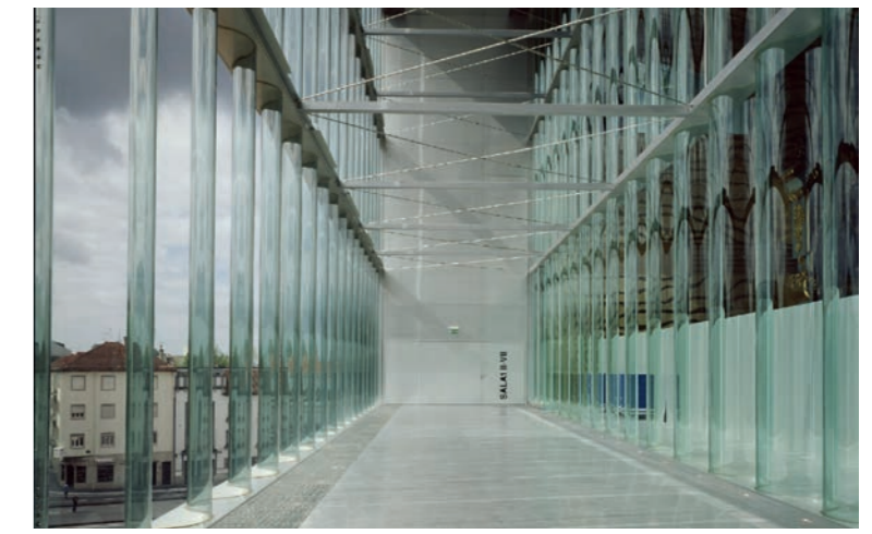
Fig. 22: Photograph of Casa da Musica twin facade access hall. Image by Philippe Ruault
