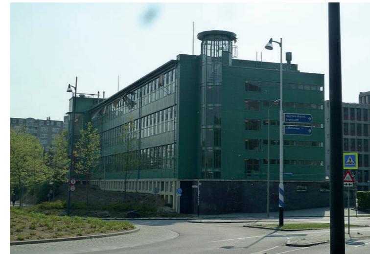
Fig. 26: Oranje-Nassau after the restoration with its original green colour
