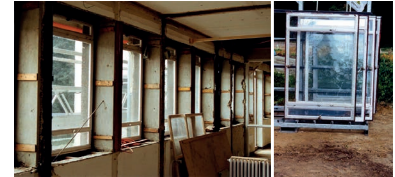
Fig. 27/28: easy removal of window frames in the Retraite
