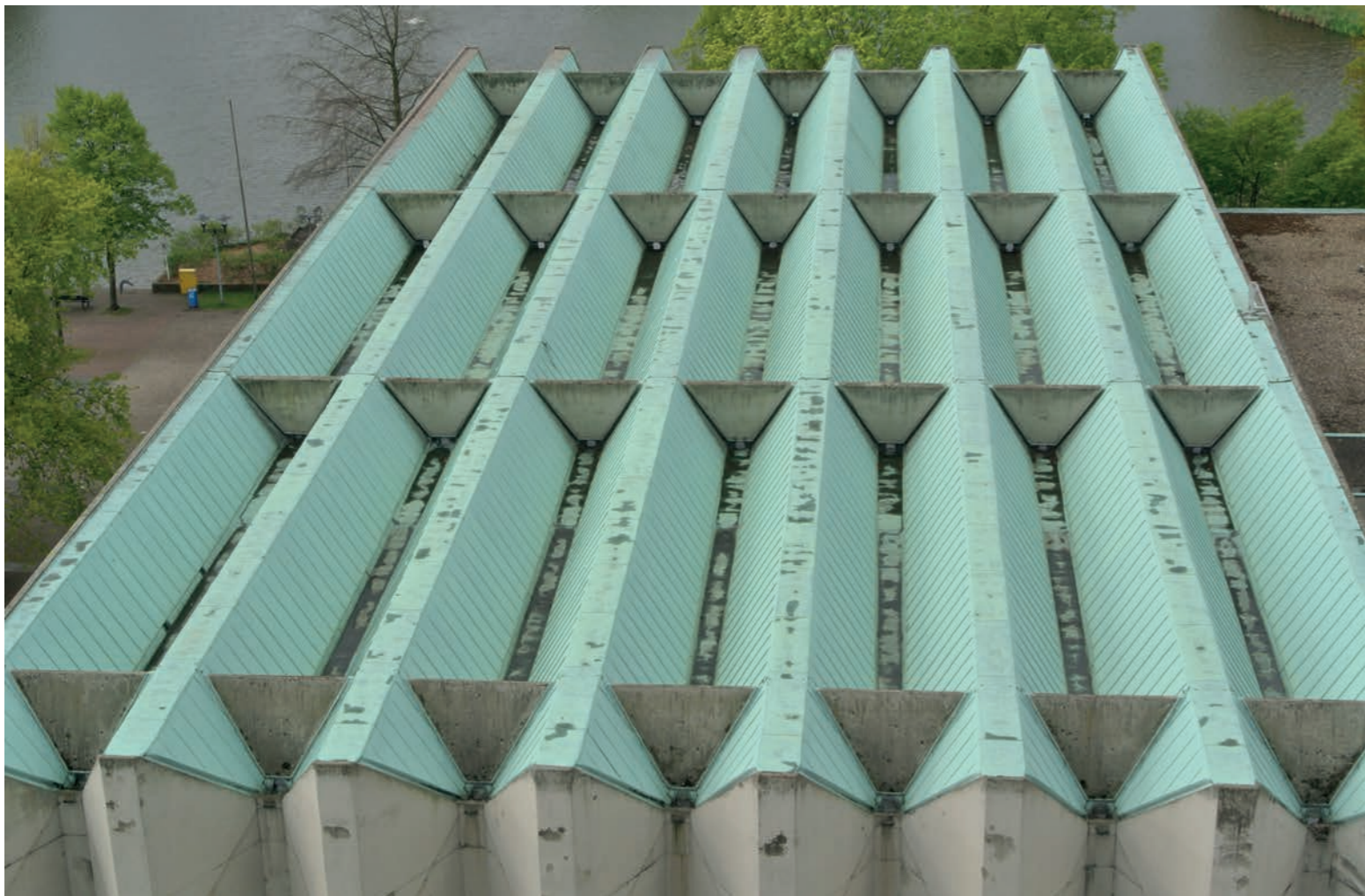
Fig. 1: Marl Town Hall, construction experiments
