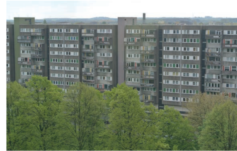
Fig. 3: Marl large scale Social housing blocks
