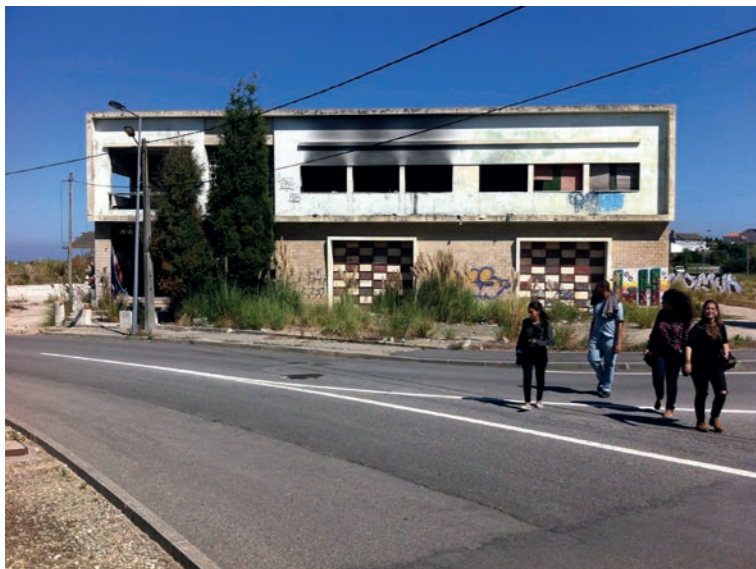
Fig. 2 Front façade of Vitasal, designed in 1955 by Eng. Elísio Souto Moura. Photo by Gonçalo Canto Moniz
