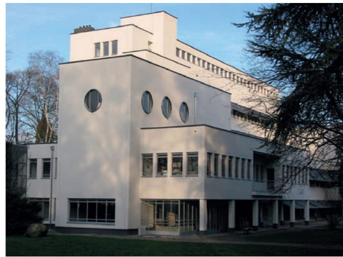
Fig. 29/30: Retraite before and after restauration
