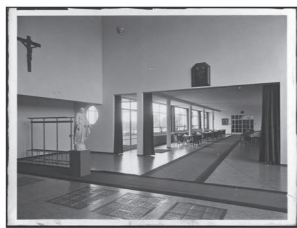
Fig. 17/18: spatial sequence in the Retraite, entrance, stairs, hall, 'veranda'
