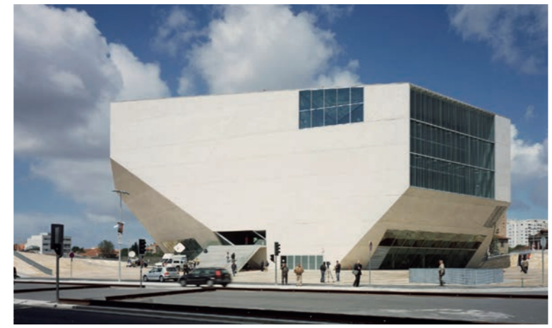
Fig. 18: Photograph of Casa da Musica exterior view from street. Image by Philippe Ruault
