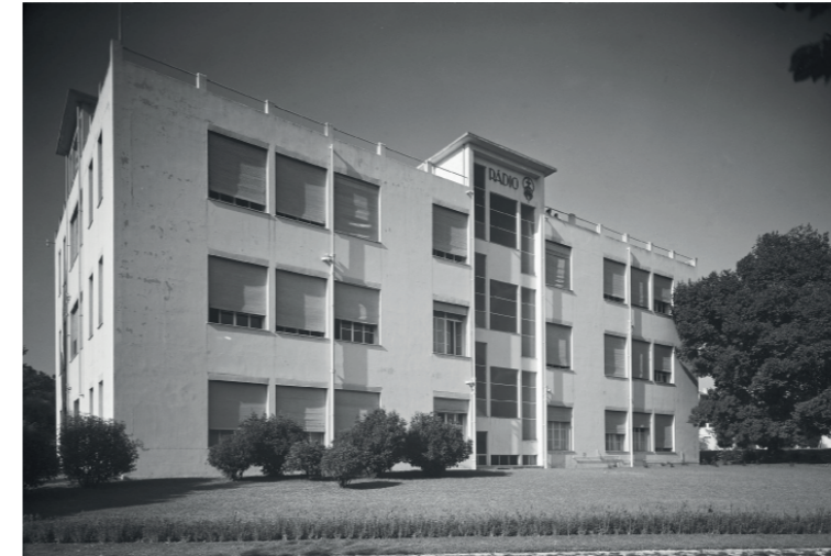
Fig. 2: Carlos Ramos. Radium Pavilion. Portuguese Institute of Oncology. Lisbon. Portugal. 1933. Southeast façade. © Art Library of Calouste Gulbenkian Foundation, Photo Mário Novais.
