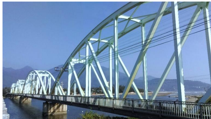
Fig. 5 – Nam O Bridge
