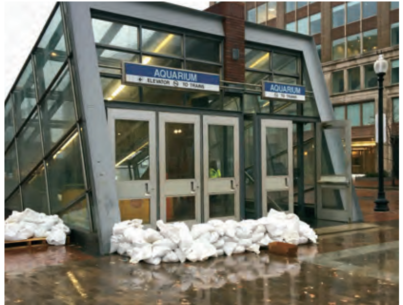
Flooding at the MBTA Aquarium Station in downtown Boston, March 2018.
