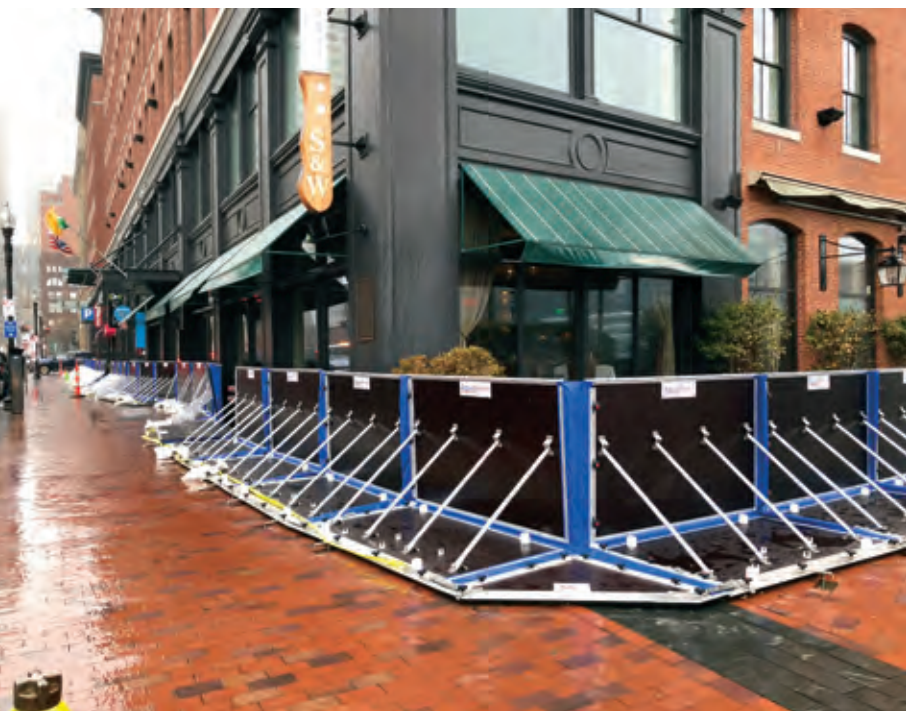
Aquafence around Atlantic Wharf to protect the building from flooding during a Nor'easter, March 2018.
