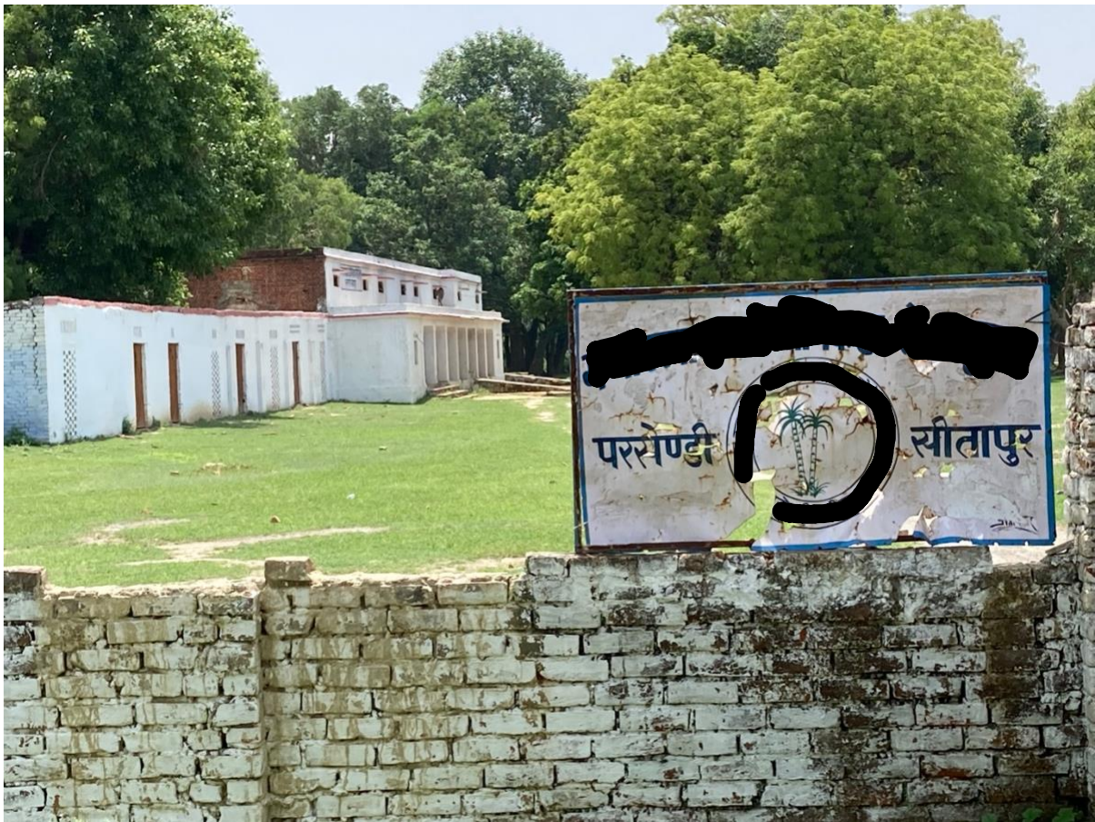
Figure 5: Boundary Wall: Village Secondary School
