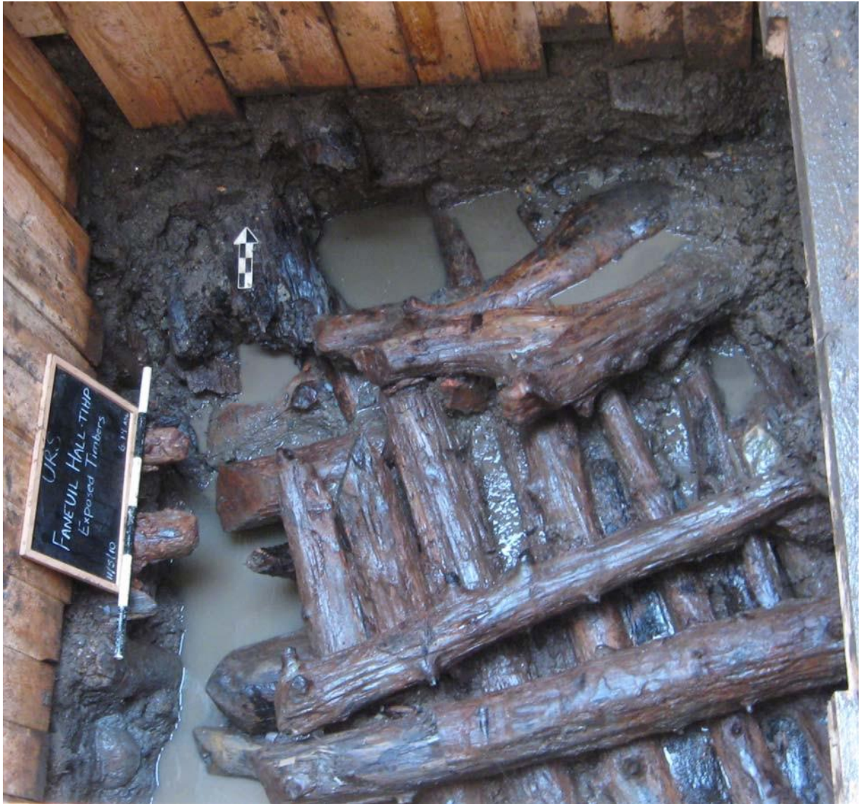
Figure 2.4. Historical grillage complex, facing North. Primary grillage is at the center of the excavation, western grillage is below the photo-chalkboard, and the north grillage is below the north arrow. From URS report, 2013.
