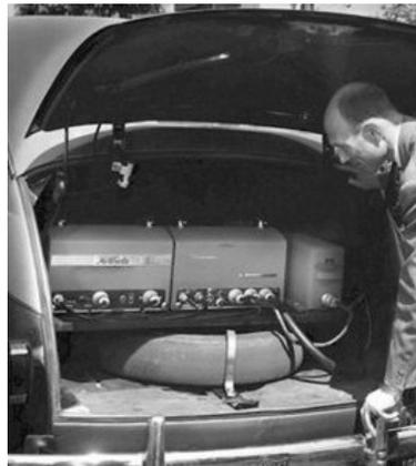
Figura 2.5: Mobile Telephone System
