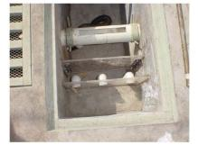
Fig. 2: Photograph that shows the details of the skimmer, oil baffle and outlet weir of the Prototype separator
