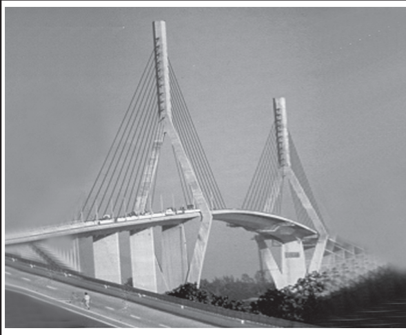
Figure 1. General view of Tampico bridge.
