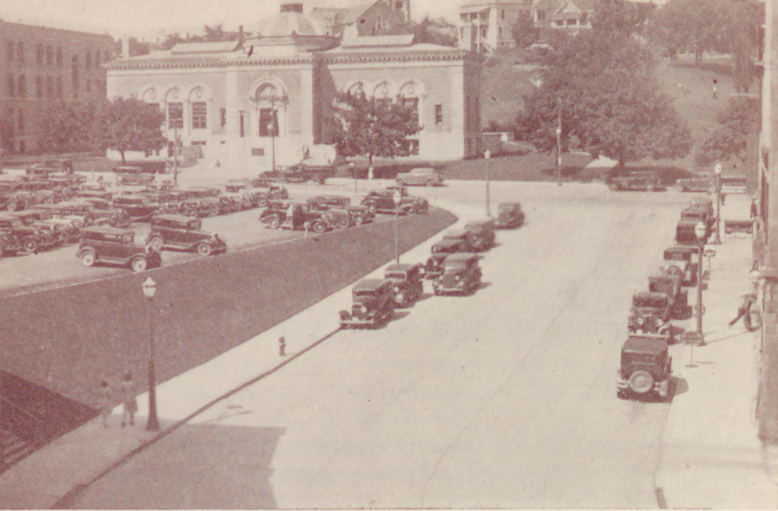
Franklin St. Looking Toward Library and Municipal Auto Parking Place
