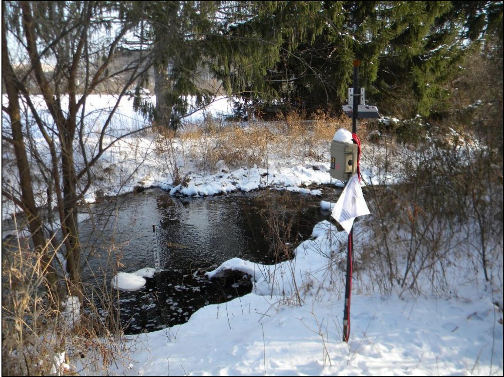
FIGURE 3: Photos of the SCCC sensor station and the SCCC stormwater pipes that discharge at the sensor
