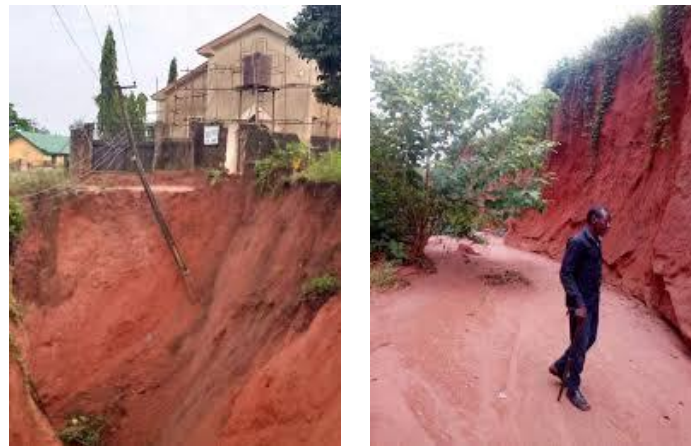
(b) Environmental destruction site through slope failure due to erosion in Umunwanwa, Abia State, Nigeria
