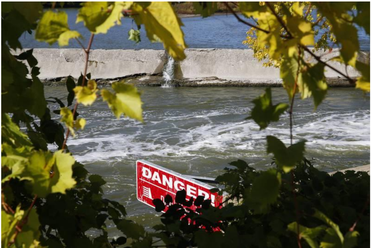
Figure 32 Danger sign at Batavia Dam (2020). Source: Chicago Tribune
