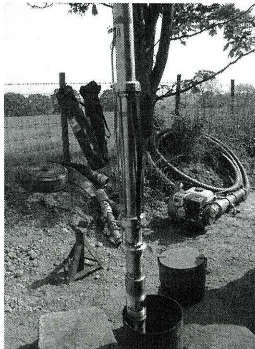
Figure 9.9: The Langwathby borehole with a camera sonde.
