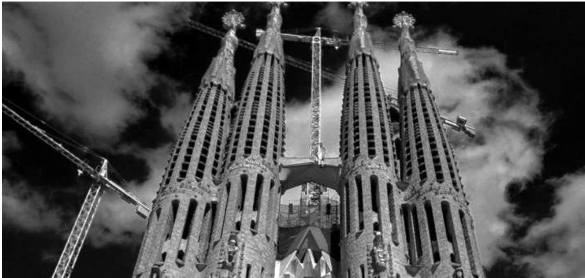
Figure 6: Sagrada Família , by Antonio Gaudi. The design complexity was achieved with the idea of parabolic and hyperboloid without the aid of any parametric software Source: https://www.flickr.com/photos/11266811
