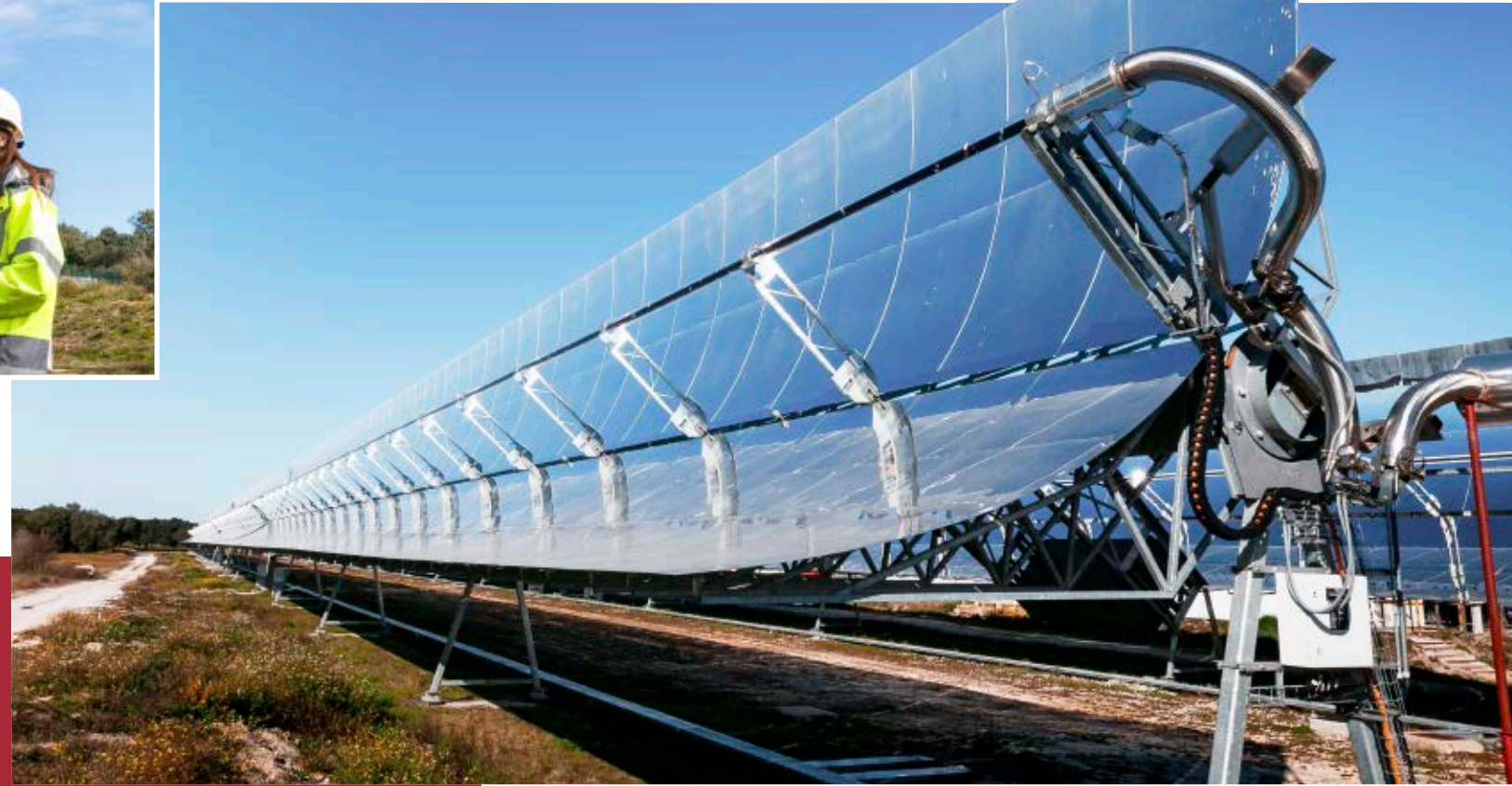
In the test facility, molten salt flowing through the metal pipe in the middle of the parabolic reflector is heated by solar radiation.
