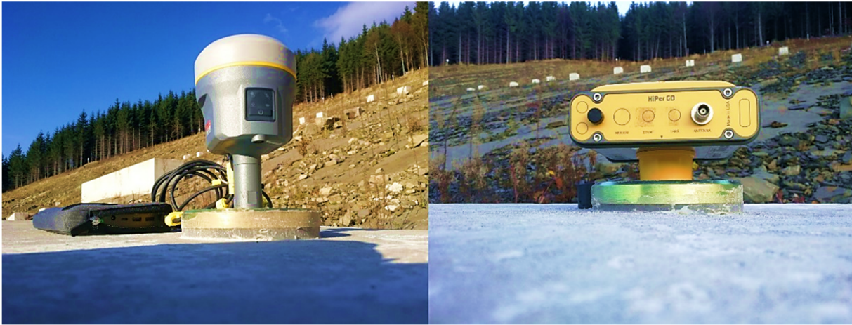
Fig. 2 GNSS receiver Trimble R10 (left) and TOPCON Hiper GD (right) stabilized at established monitoring points.
