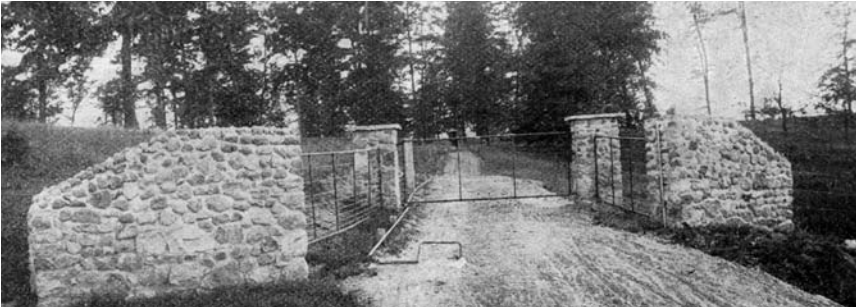
The entrance lane to Virginia Meredith's Norborough Farm in Cambridge City, Ind. The device in the lane would automatically unlock the gate when her carriage crossed over it. Reproduced from Dignam's Magazine .
