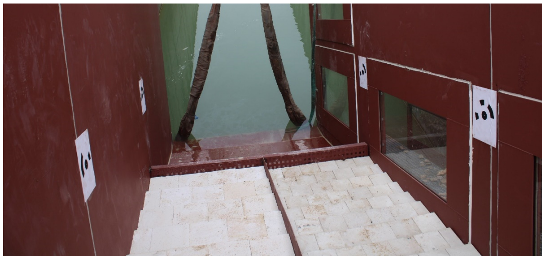
Figure 23. Detail of the perforated metal plate, where the downstream row of the WSB was supported.
