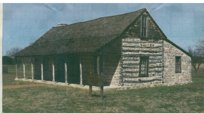
"The Material Culture of German Texans" photos The Heinrich and Johanne Lindig house, built about 1877, is a double-pen log house with a dogtrot. It was built in the Pedernales settlement, which is near Stonewall.
