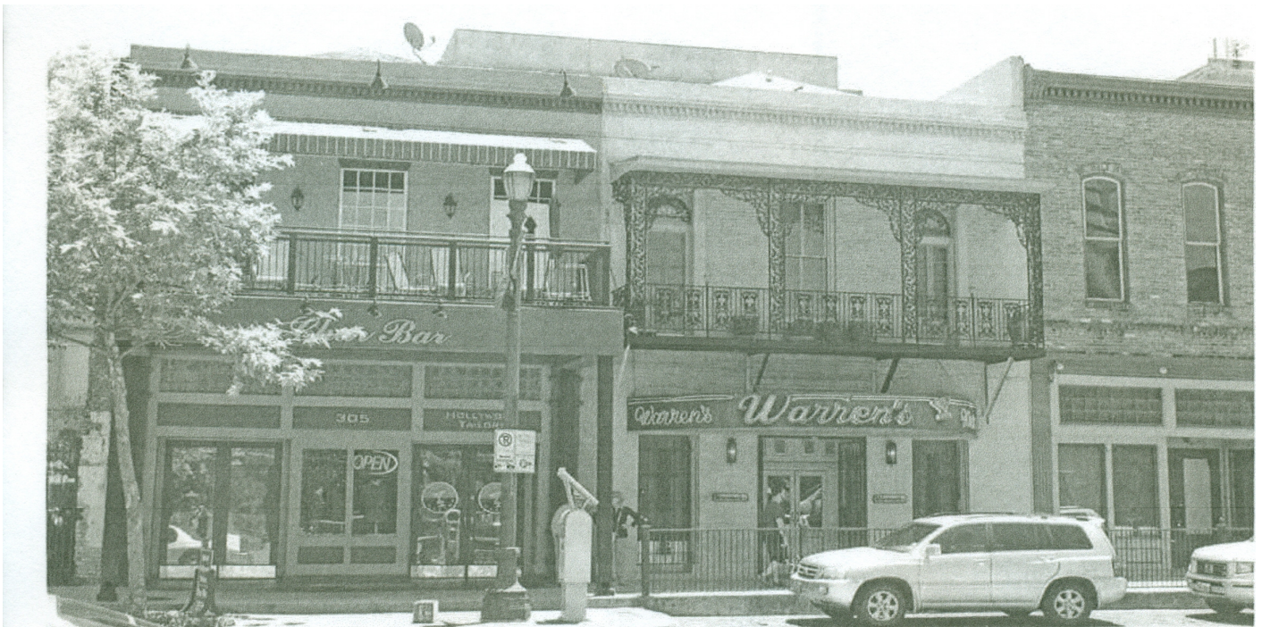
The Fox-Kuhlmann Building, completed in 1866 at 305-307 Travis Street, is a City of Houston Protected Landmark.
