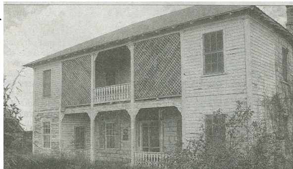
William Pfluger finished building his home in 1875. The family sold it in the 1990s, and it has since had problems with rotting and decaying wood.
