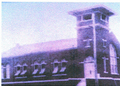
Pictured above is Saint Paul’s original building as it stood in 1912.
