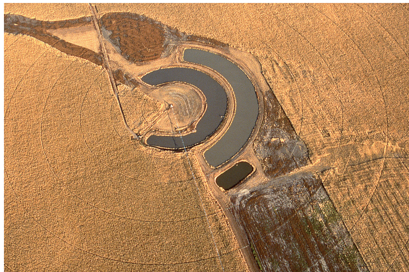
Nebraska has more acres of wetlands than any surrounding state, due in large part to the extensive wetlands remaining in the Sandhills. However, in many parts of the state, wetlands have been destroyed or highly altered. Pictured here is the location of a historic Rainwater Basin wetland. The once shallow and productive wetland has been drained into deep pits that were excavated to concentrate the water and to allow for the passage of a center-pivot irrigation system. JON FARRAR, NEBRASKALAND
