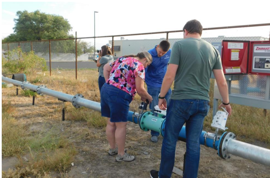
Academy participants examining water technology at the Middle Niobrara NRD demonstration and training facility.
