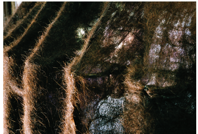
11 Pavilion exterior with hair and steel sub structure. (2019, Visut Innadda).
