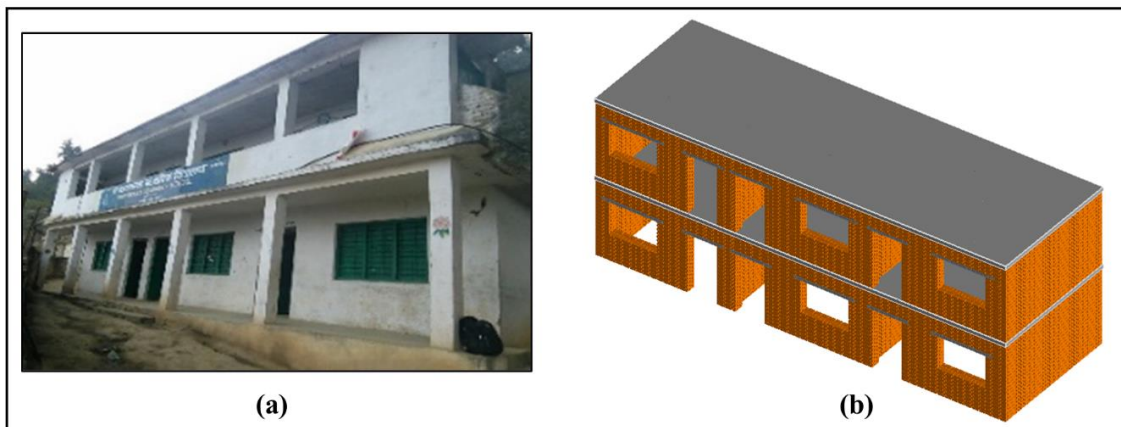
Figure 13. URM7/MR/LD building: (a) isometric view and (b) AEM numerical model.
