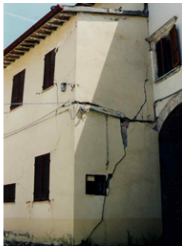
Figure D.13. Typical two-storey masonry building in Nocera Umbra, Italy
