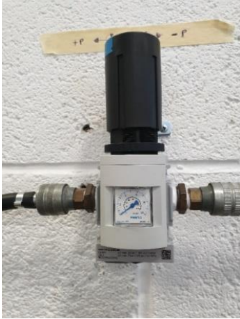
Figure 3.10 Photo of the air flowrate regulator
