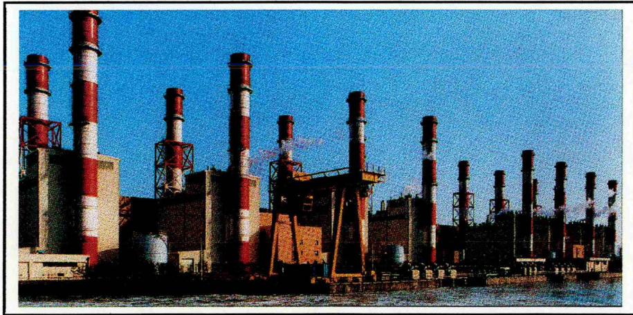
Figure 21: Seoinchon Combined Cycle Plant
