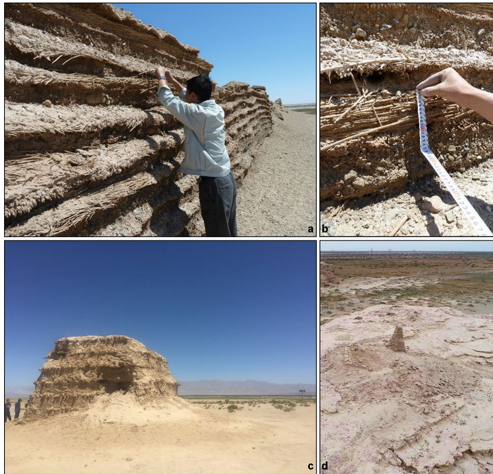
Figure 2. Remnant wall segments and beacon towers of northwestern China. (a) Sampling of Phragmites culms from a wall section at Majuanwan (Site 7); (b) Reed fascines alternating with layers of rammed earth at Majuanwan. Near center is a fascine of Phragmites culms that were sampled for analysis; (c) Remnants of Sishilidadun Beacon Tower (Site 14) dating to the Song Dynasty. Although not visible, the beacon tower was constructed like the wall section in panel a, with rammed earth alternating with reed fascines; (d) Low altitude air photo of the Yakelun Beacon Tower (Site 11), courtesy of Xingjun Hu. Note the wild plants growing adjacent to the tower.
