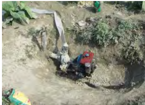
Figure 17.4. Small pump used for groundwater irrigation in northern India.
