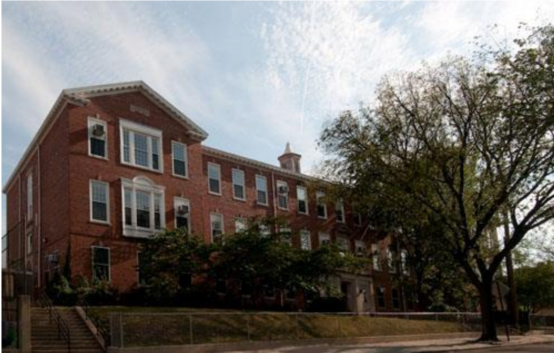
Figure 5.02 – Exterior Photo, Google Images
