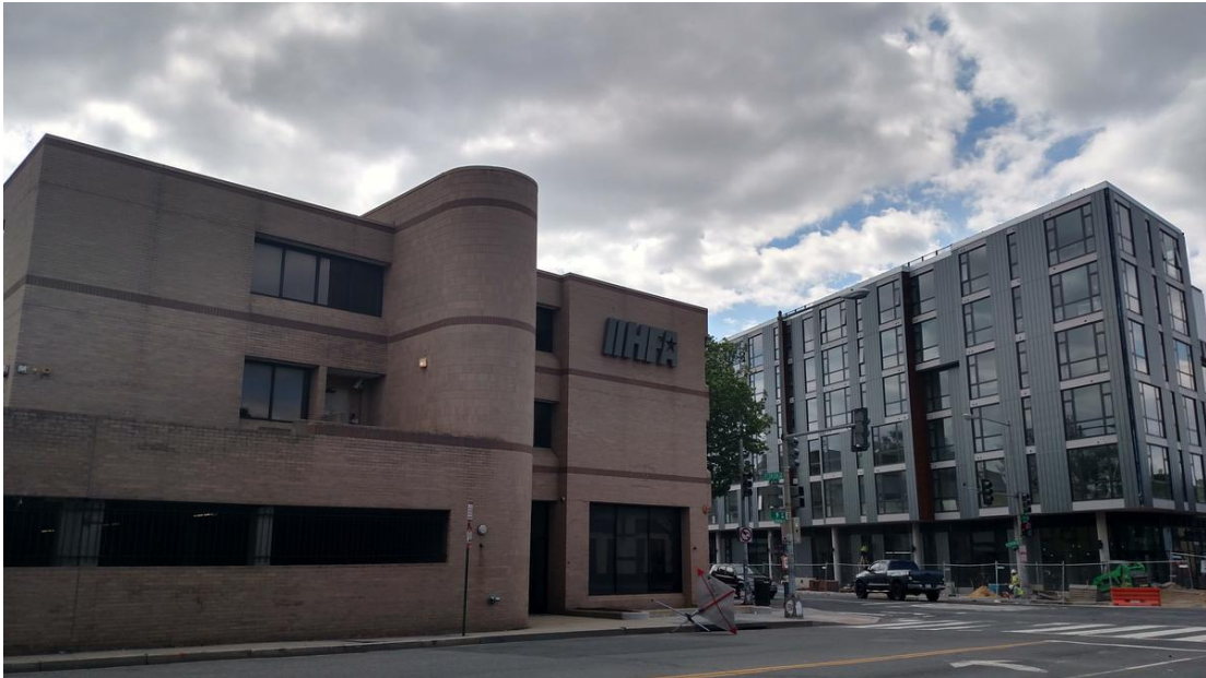
Figure 5.07 – Exterior Photo, Google Images
