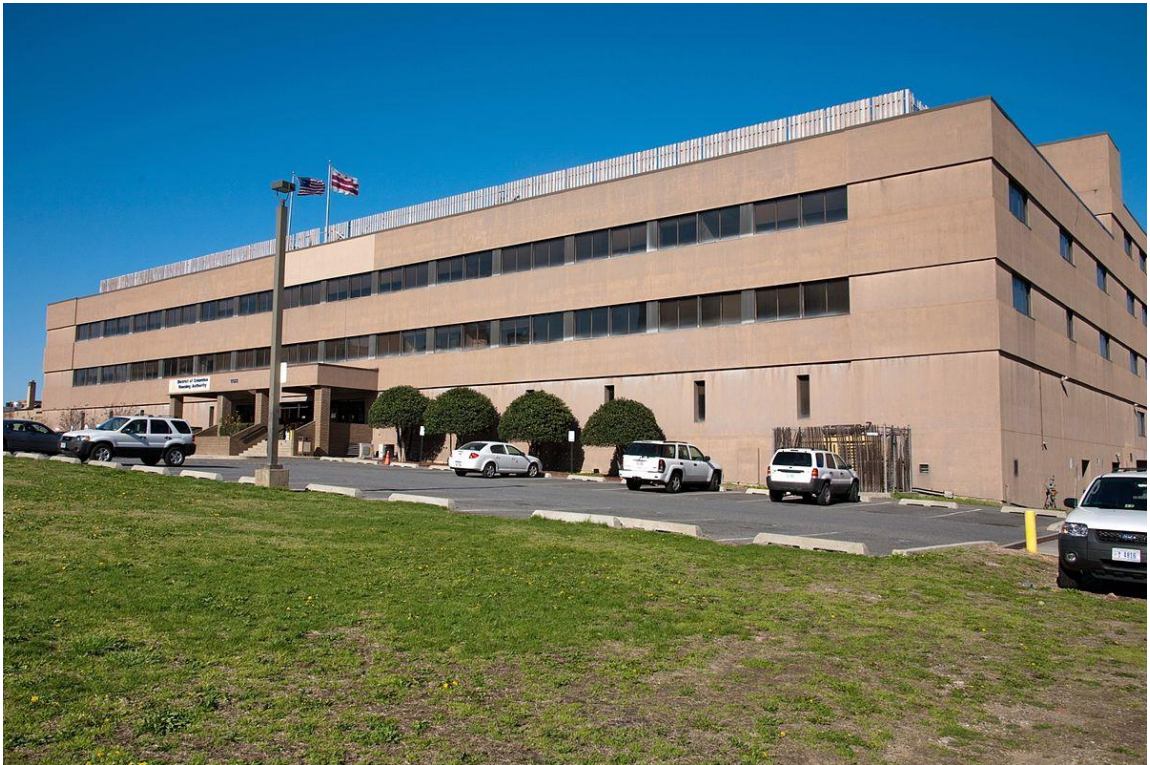
Figure 5.04 – Exterior Photo, Google Images
