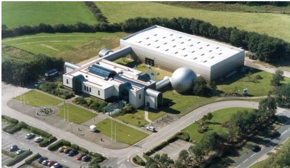
Figure 3.5: Aerial photograph of the former visitor center at the Sellafield nuclear complex. (Source: Google)
