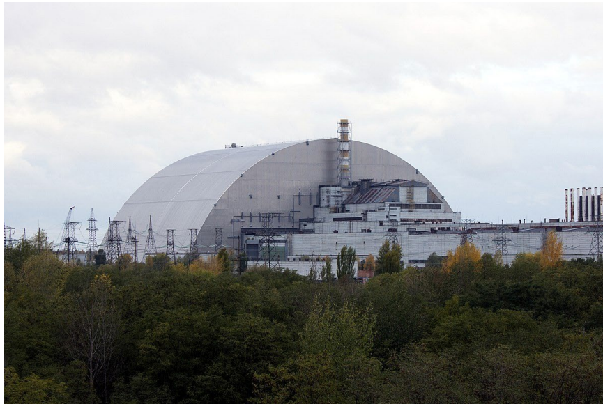
Figure 2.5: Image showing the present-day Safe Confinement Shelter covering the damaged reactor 4 at Chernobyl. (Source: Google)
