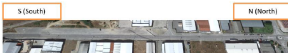
Figure 1- Test zone: 600m length and 34m maximum width. The north side is where the roundabout is (right side)
