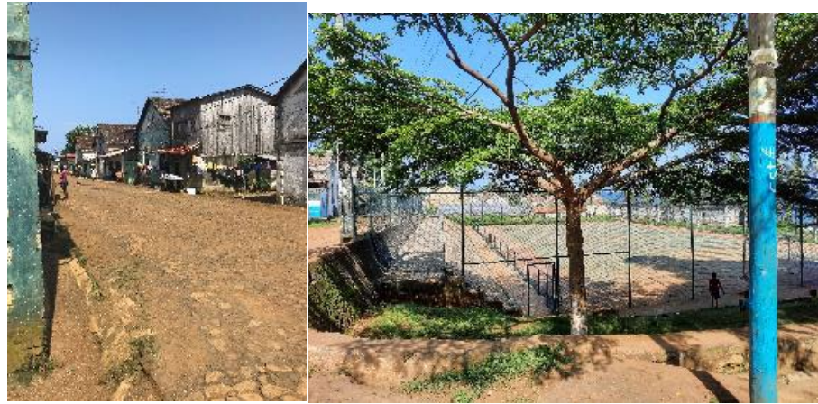
Figure 4. Present-day occupation in roça Água Izé: sanzalas and recent extensions (left) (photo by Sara Eloy); the current use of the terreiro (right) (photo by Rui Brito).
