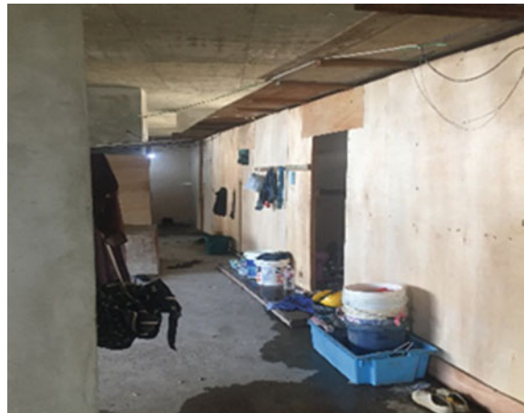
Fig. 2 Construction site A makeshift workers' quarters set-up made of plywood partition boards
