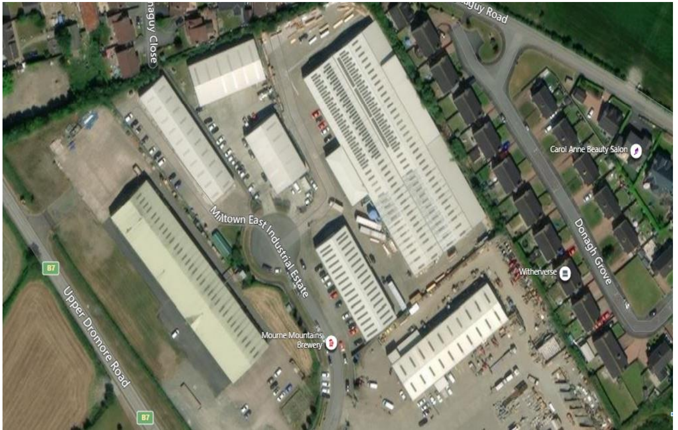
Figure 36. Examined PV arrays installed at Warrenpoint
