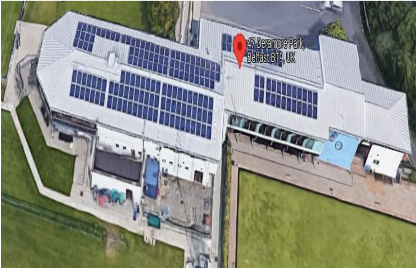
Figure 34. Examined PV arrays installed at Harlequins
