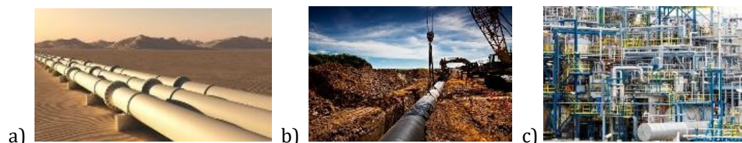
Figure 1.2: a) Over ground gas pipelines, b) underground water pipeline and c) plant pipes [4 - 6].
