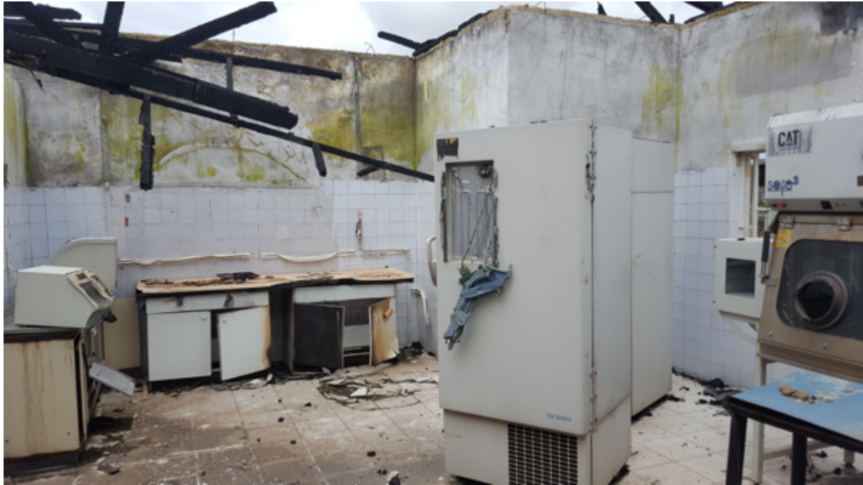
Figure B-1 The lab at the Holy Spirit Hospital following a lightning strike and lab fire in November 2016. Makeni, Bombali District, Sierra Leone. July 2017.
