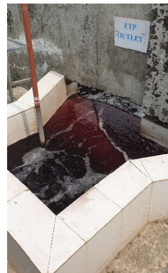
Figure 10.9 Water discharged from ETP outlet into local drainage Source: Author (2020) in field visit of case study units
