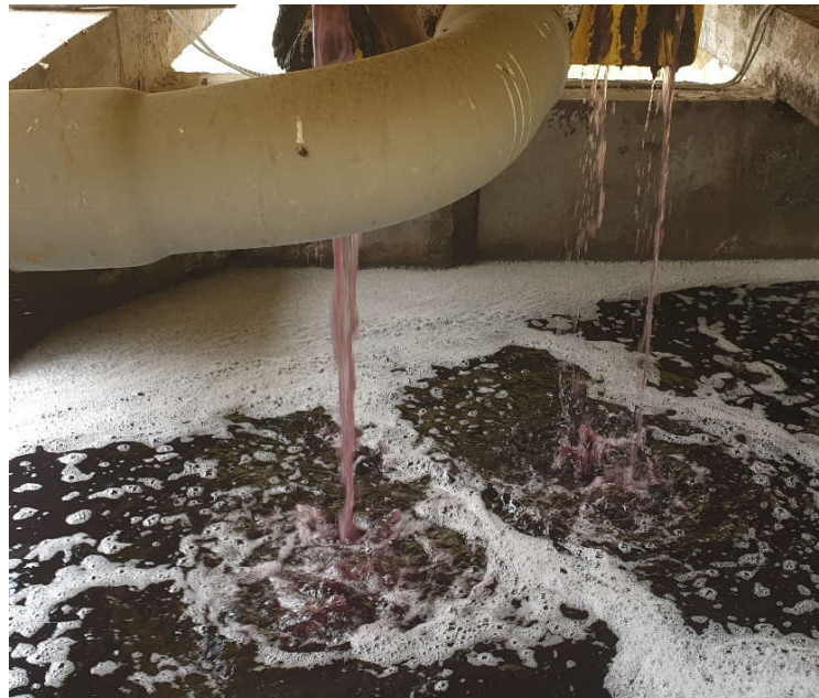
Figure 10.7 Water discharged into ETP for treatment Source: Author (2020) in field visit of case study units
