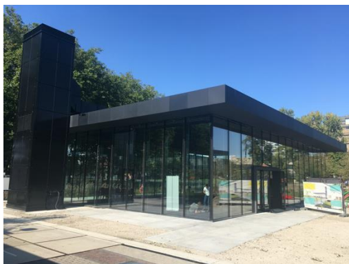
Fig. 2 – Co-Creation Center Building, located in the TUD Green Village, The Netherlands
