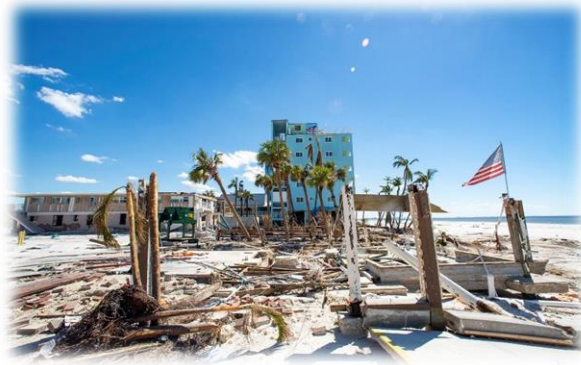
Image 3. Fort Myers Beach after Hurricane Ian, 2022
