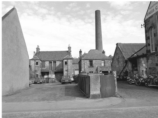
Plate 4.6 Victoria Works Chimney
