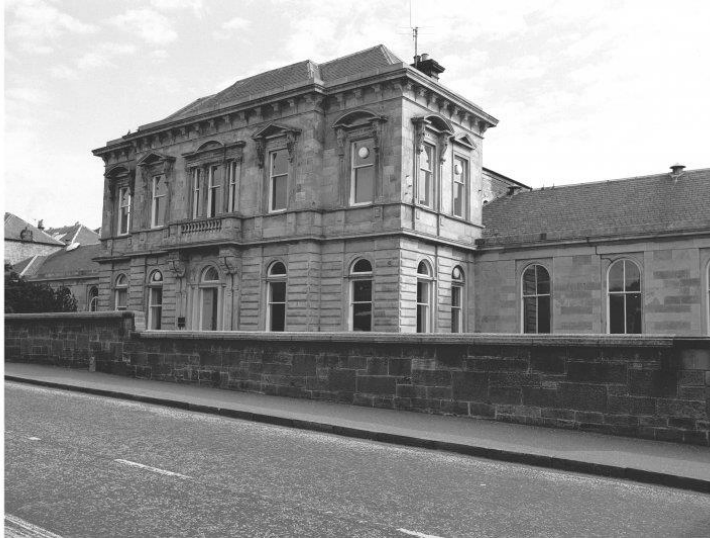
Plate 4.5 An External View of Victoria Works Administration Block owned by Inglis & Co. Designed in an Italianate style
